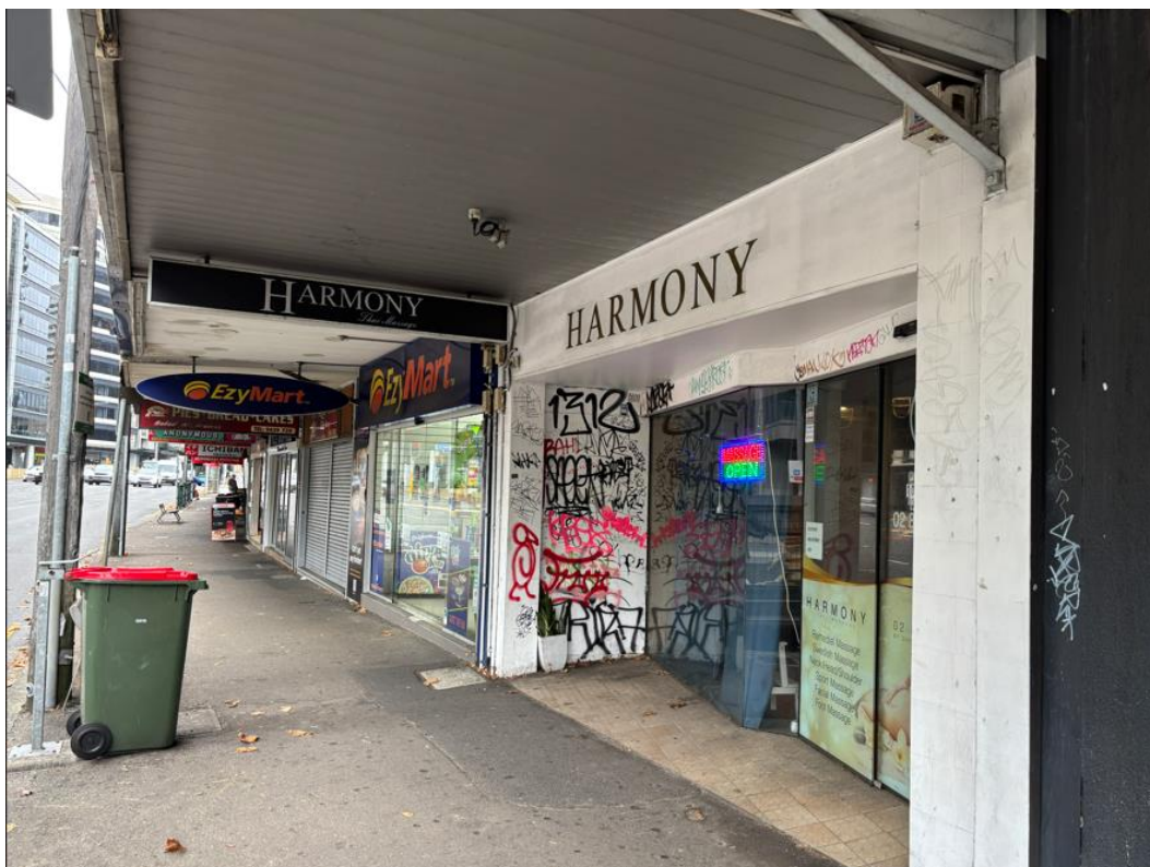
Photograph 10 View of northern entrance of the property (32 Pacific Highway).
