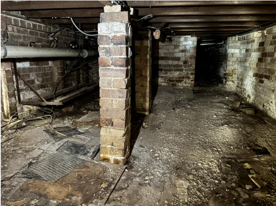
Photograph 3 View of crawl space (28 Pacific Highway)
