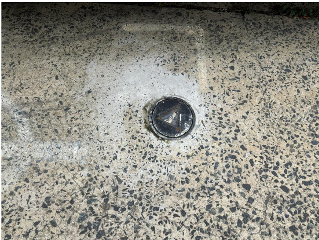
Photograph 6 Previous monitoring well location (JK, 2025) (28 Pacific Highway)
