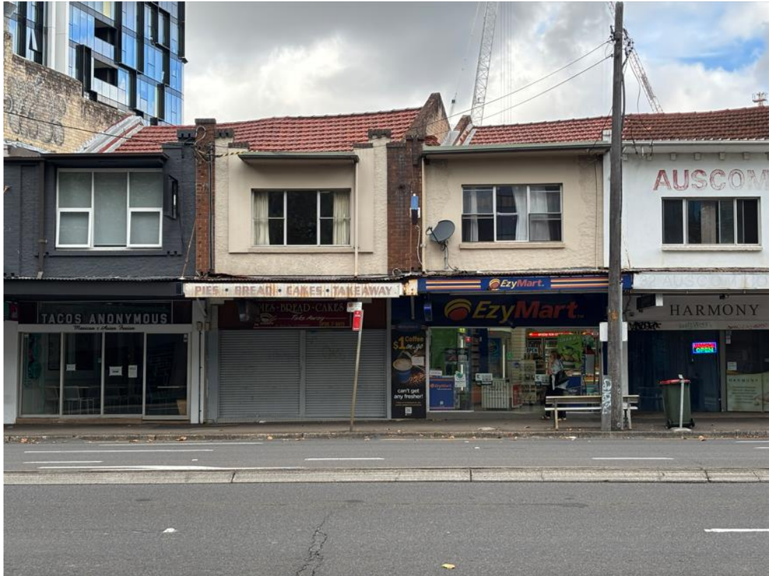
Photograph 1 View of two storey commercial building located at 28-32 Pacific Highway, Looking south.
