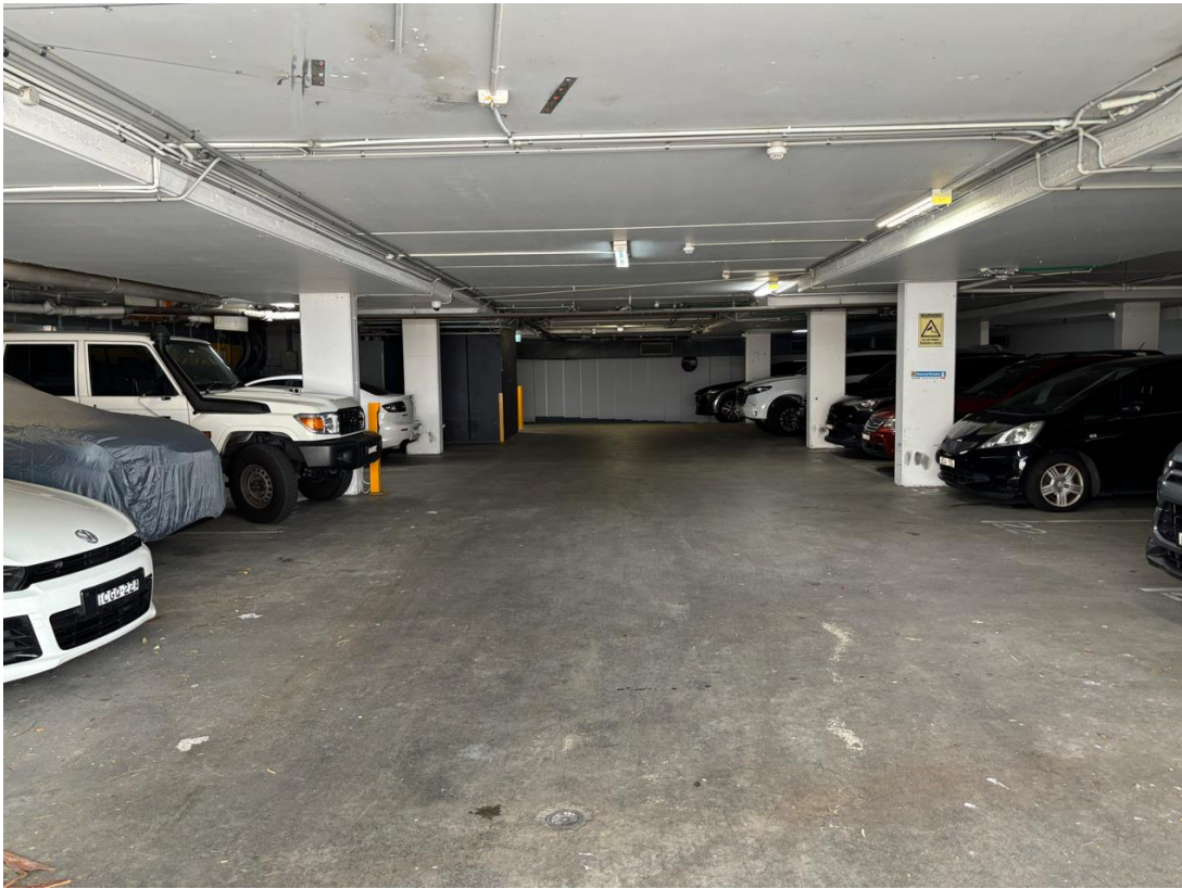
Photograph 17 Concrete floor within basement (34-38 Pacific Highway).
