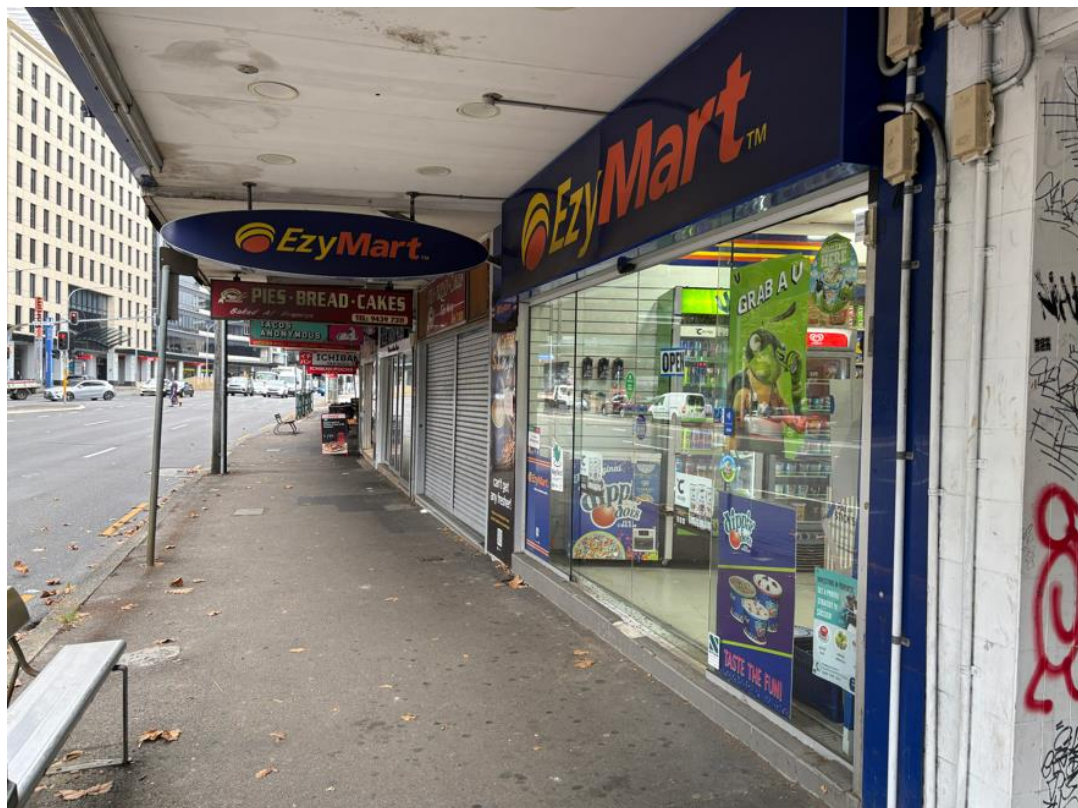
Photograph 8 View of northern entrance of the commercial building (Ground level), looking east.
