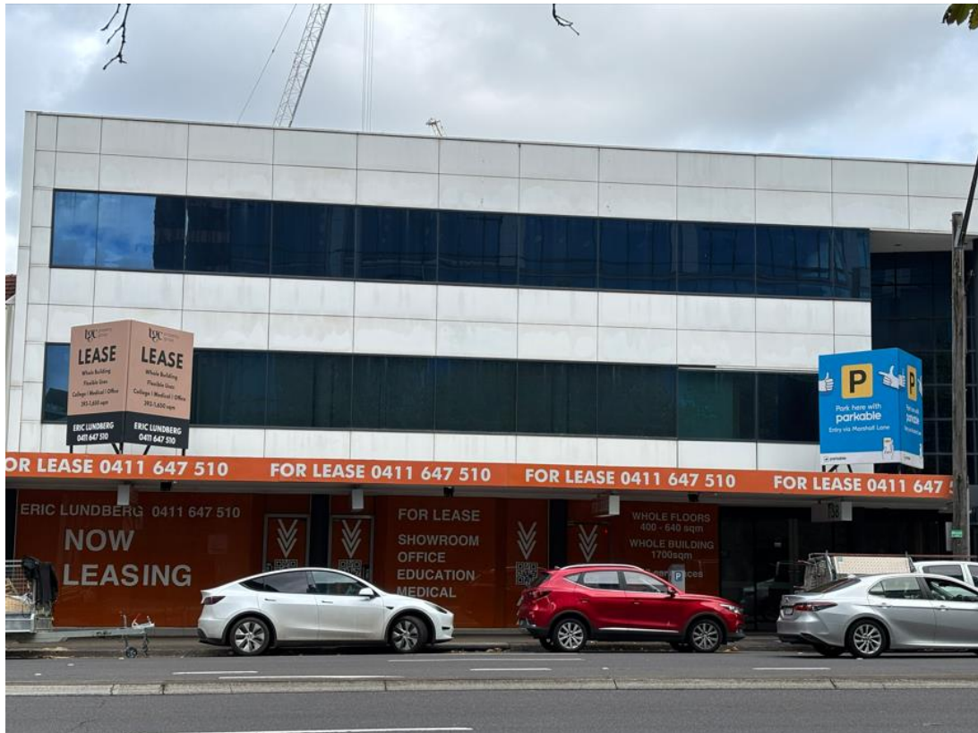
Photograph 11 View of three storey commercial building at 34-38 Pacific Highway.
