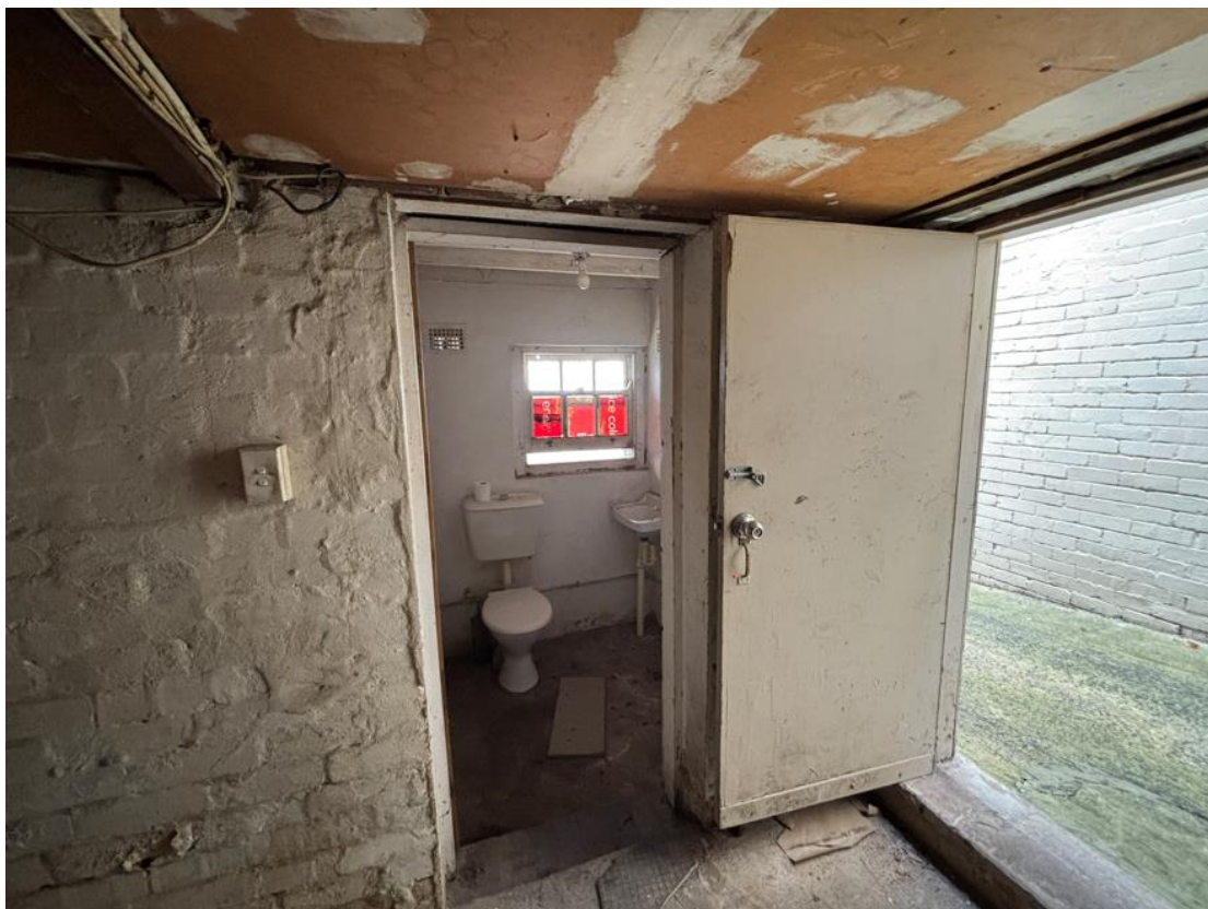
Photograph 5 View of toilet in the lower ground level (28 Pacific Highway).
