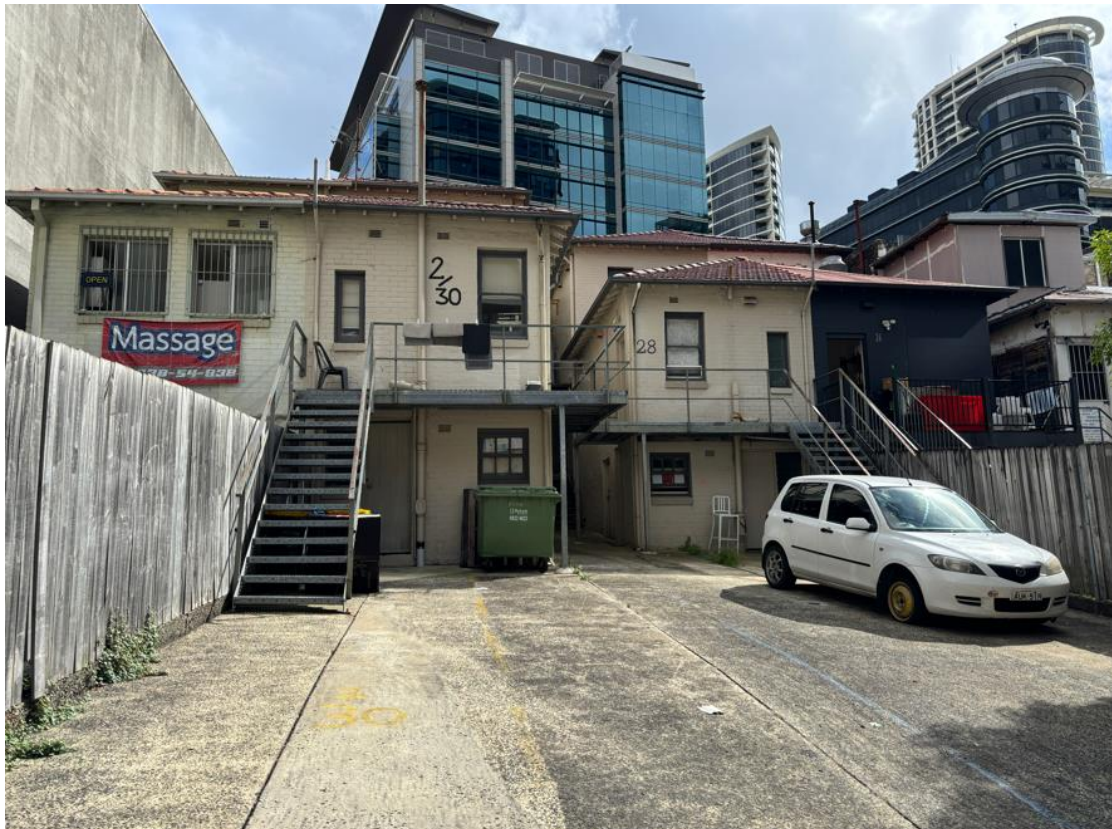
Photograph 2 View of residential building located at 28-30 Pacific Highway, Looking north.
